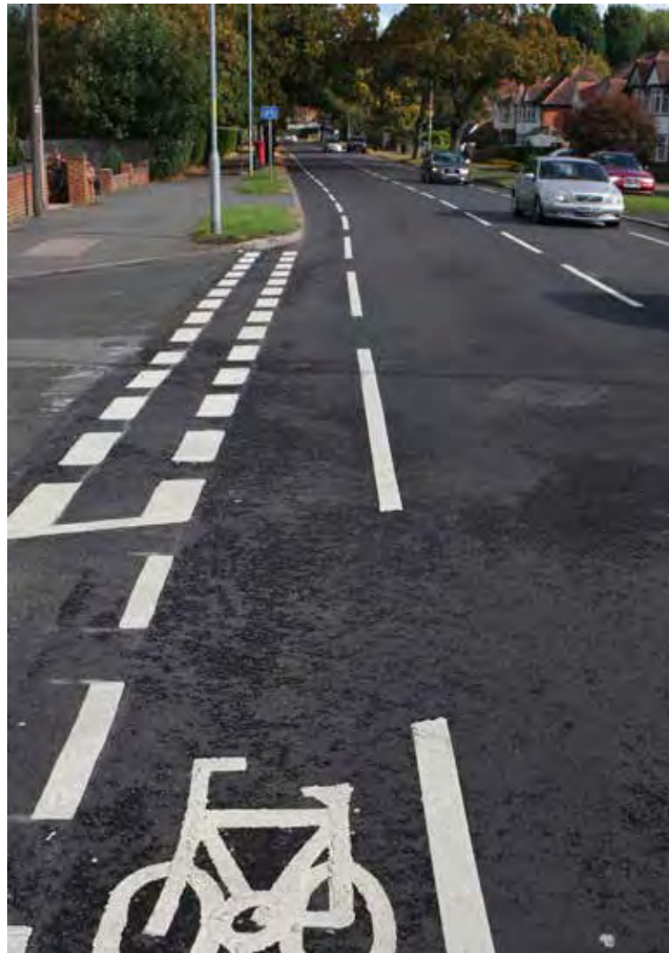
On-road national cycle route on Bromsgrove Road
