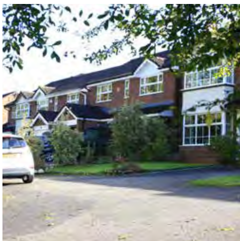
Facade materials largely comprise render and brick
