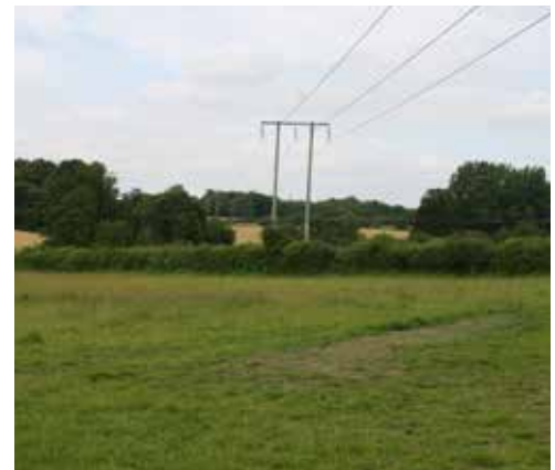
Existing overhead powerlines cross through the site
